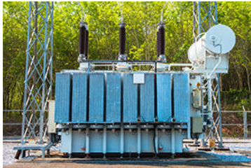
STO-50 is a 100% PDMS silicone oil formulated for use in liquid filled transformers.
